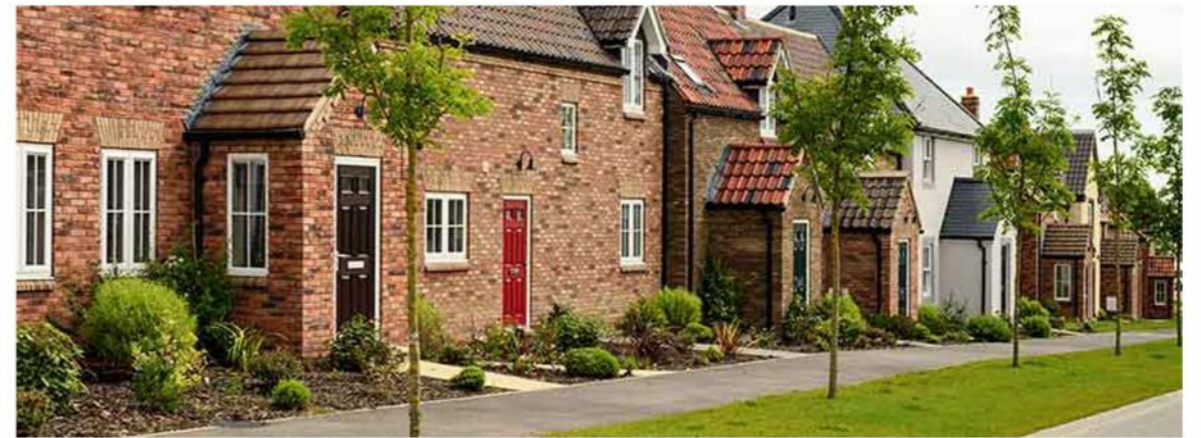
Traditional housing designs with high quality materials along a verdant street
